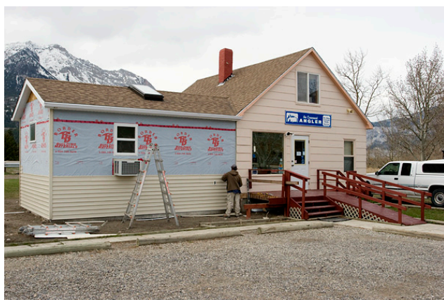
Putting up siding on the new addition
